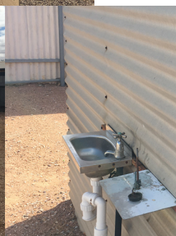
Wash basin located outside toilets
