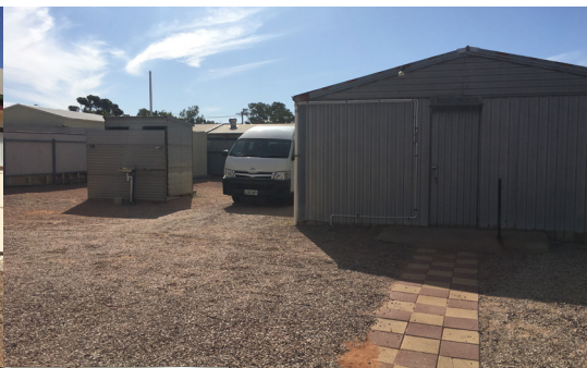
Current hall and toilets - the hall is a shed
